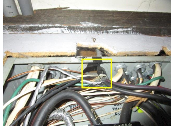
Electrical: Missing bushing or strain relief clamp
