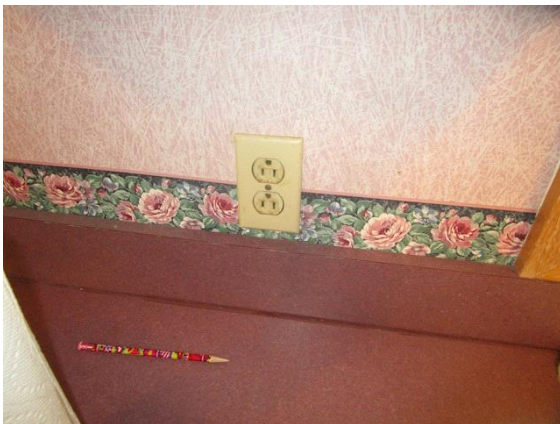
Electrical: Kitchen - not GFCI
