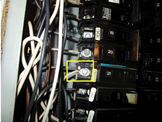
Electrical: Double tapped breaker
