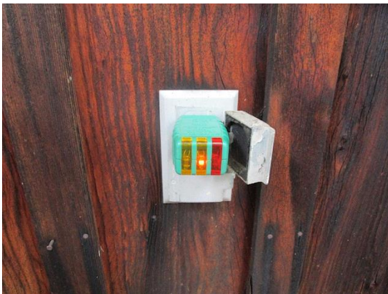
Electrical: Basement - ungrounded
