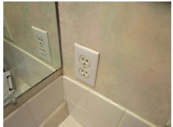
Electrical: Hall bathroom - not GFCI
