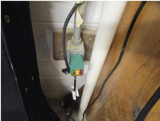
Electrical: Unfinished basement - ungrounded and not GFCI
